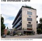
Le Corbusier demonstrated his principles of orefabricated and . standardized plan and structure. This was the first building that used steel frames for windows and
